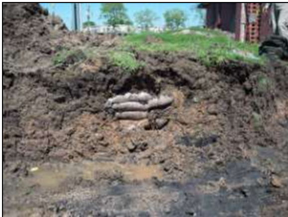
Figure 9. North profile of generator pad site showing the undisturbed Lake Charles clay at the base of the pit and sandbags and PVC pipe in the wall. The sandbags and PVC pipe were placed in the trench that brings electrical conduit to the generator pad site.
